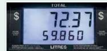
Display panel at Petrol Kiosk
